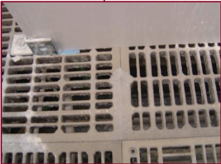
*Figure 6 – Floor grate adjacent to tool after cleaning. Much residue removed, but additional cleaning applications will be required.*
